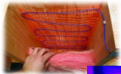
Heatweave® electric mats staple-up between joists. Note the insulation below the suspended mat.
