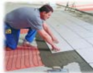
HeatWeave taped to a slab and covered with thin-set masonry and tile.
