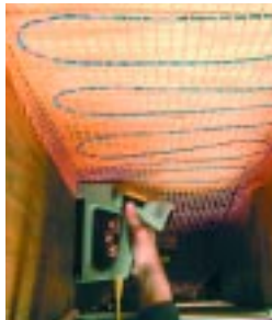
Heatweave® electric mats staple-up between joists. Note the insulation below the suspended mat.
