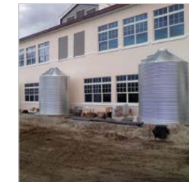
Water Storage Tanks
