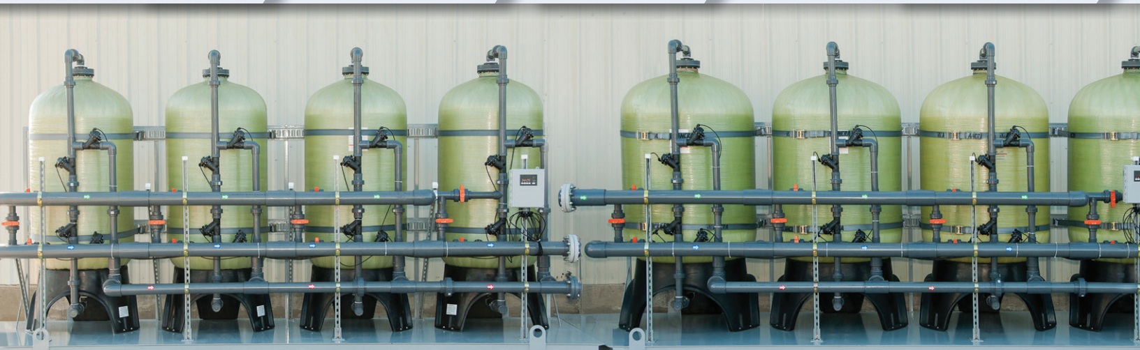
Parallel 36" x 72" Quad Micro Z Filter System
