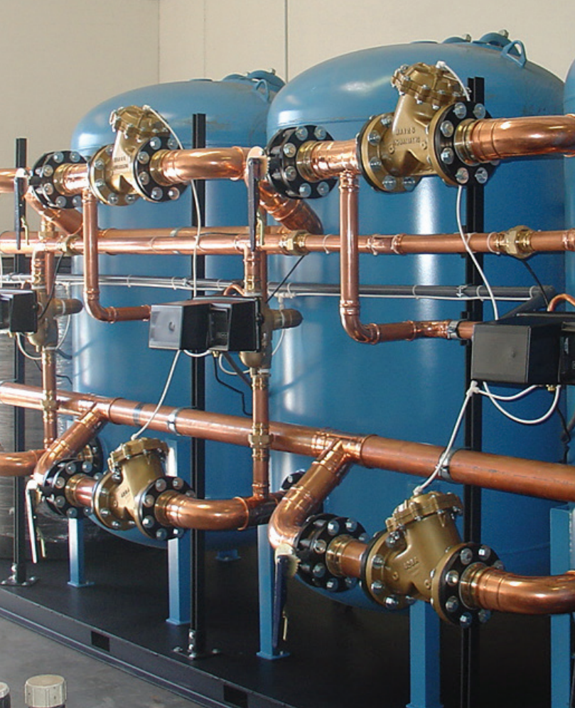
System Shown with Optional ProPress® Fittings
