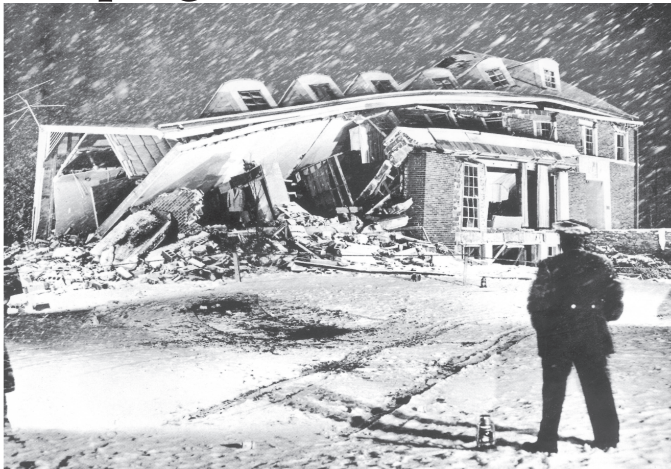
Seven persons were hurt in water heater explosion at fraternity house.
